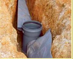
PACDRAIN and ROADRAIN water drainage and collection solutions. They have an waterproofed core, blocking any sideways water movement. Their void ratio is higher than drainage ditches (French Trench): 0.9 compared to 0.2.
